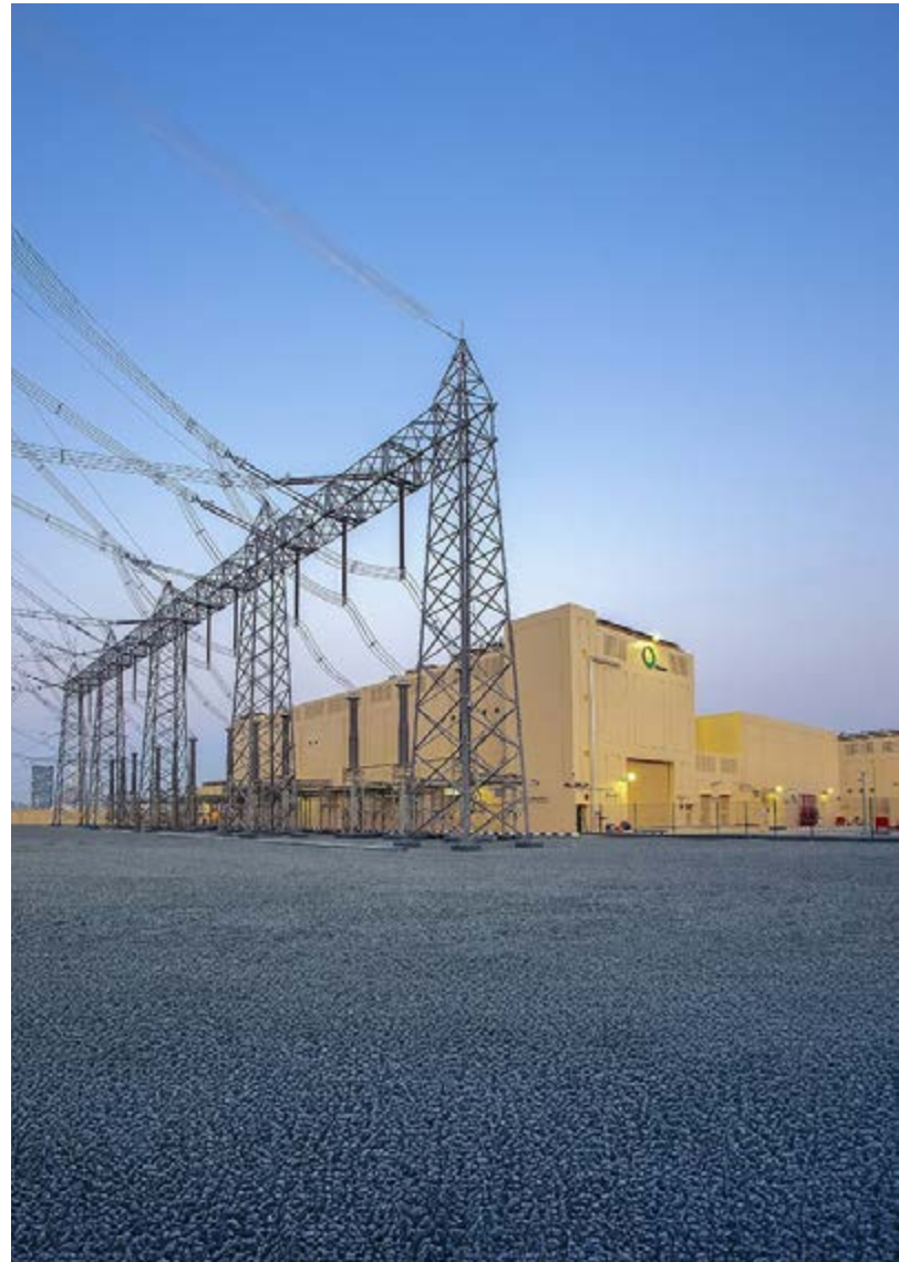
Figure 2. The DEWA Canal Garden Substation, a 400/132 kV facility in Dubai's Discovery Garden area, was built for Dubai Expo 2020. With a capacity of 2000 MVA, it eases load on nearby areas and supports future growth. GE Vernova led the project, with Aztec Middle East handling civil works. Managed by DEWA, the substation aligns with DEWA's clean energy strategy, incorporating advanced grid technologies to drive Dubai's transition to a sustainable energy future.
